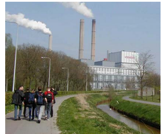
Amer power plant of Essent 1245 MWe (net) and 600 MW th pulverised coal fired 2 CHP units AMER-8 and AMER-9
