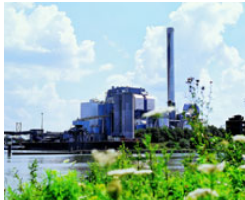
Gelderland power plant of Electrabel 602 MWe (net) pulverised coal fired ST: 180 bar, 540°C -> 0.04 bar, 30°C
