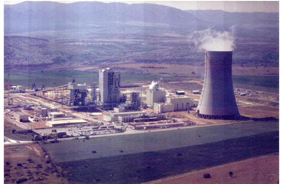
Elcogas Puertollano plant (ES): 320 MW e
